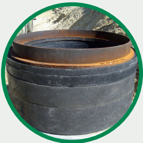
Ø600 well raised with riser rings and fixed frame
